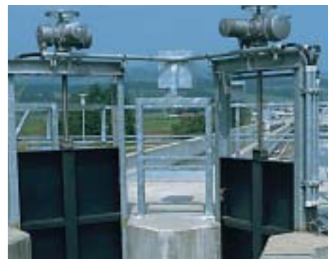
WAGO PRO slide from ERHARD ARMATUREN. TECADUR PET combines outstanding sliding properties with low moisture absorption and high dimensional stability.
